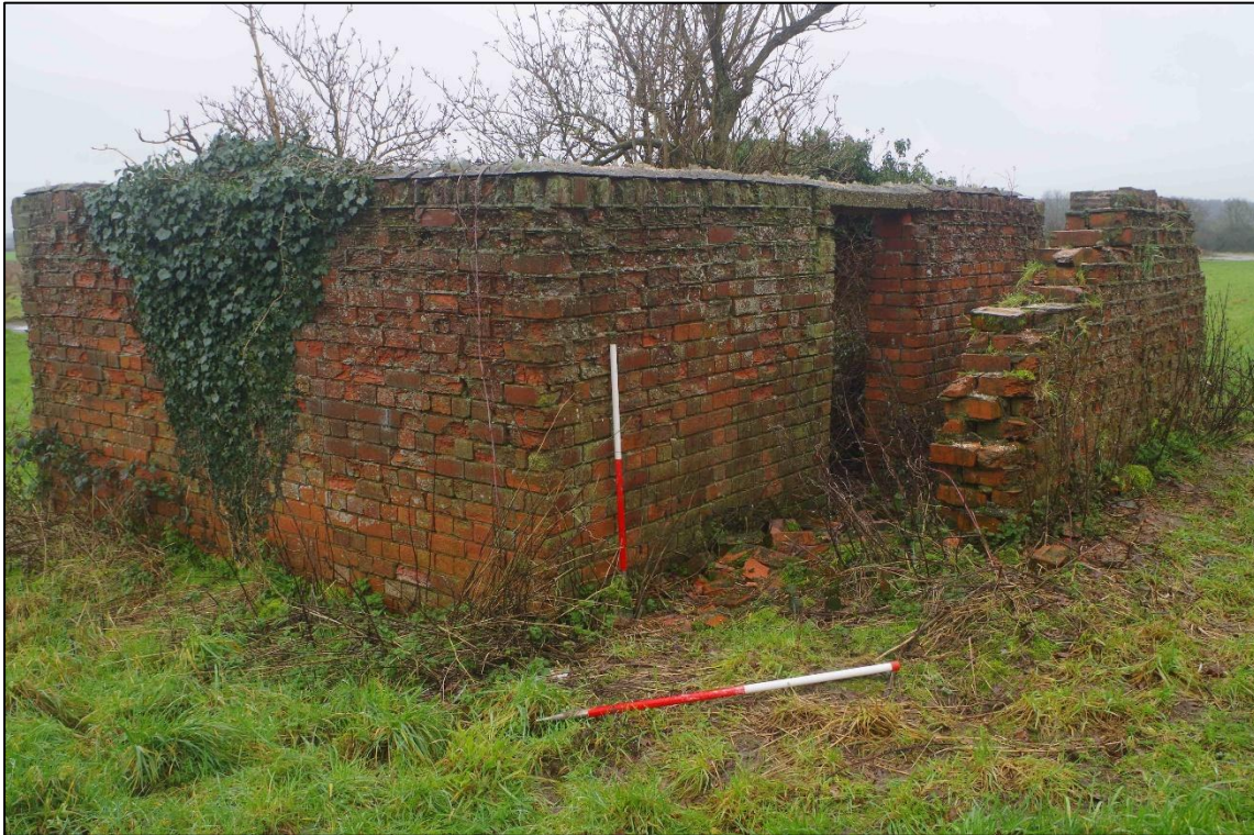
Plate 6) View of the M&E Plinth building, facing north
